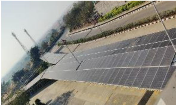
❖ Solar Panel Installation on Carport Roof :
