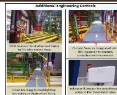
Access Control & Floor Marking in Warehouse
