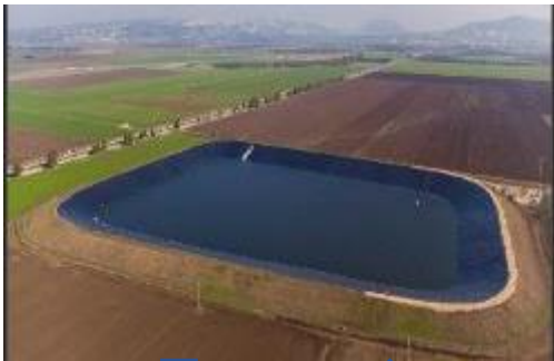
Rain-Water Harvesting Lake @ PCP1 (1000 KL)
