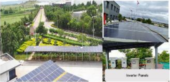
❖ Solar Panel Installation on Pedestrian Walkway Area :
